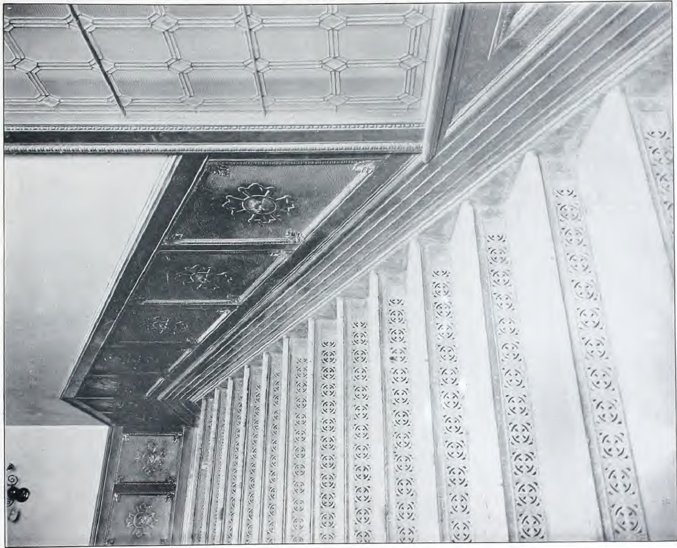
Fig. 148. —Interior View, Temple Building, Toronto.
